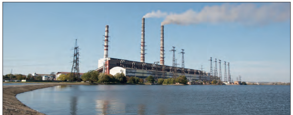
► Burshtyn Thermal Power Plant
